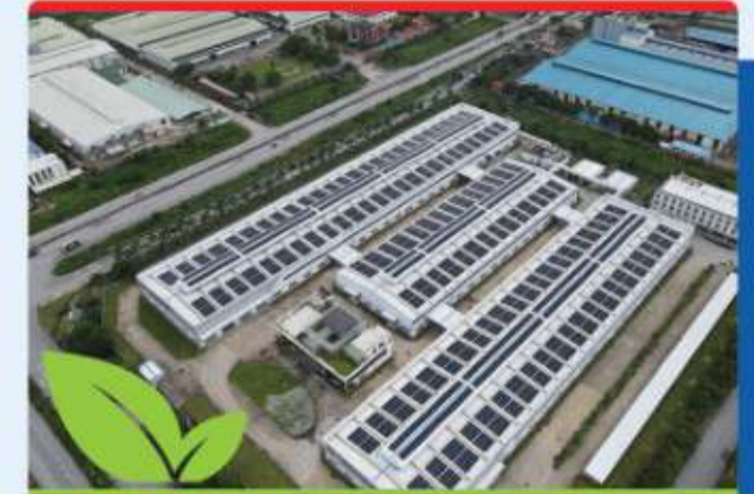
Tran Phu Wire & Cable Project
