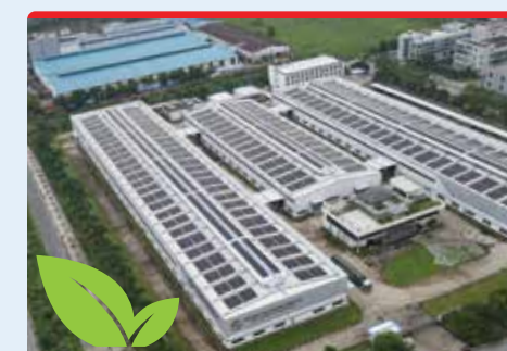
Tran Phu Electric Cable Factory Project
