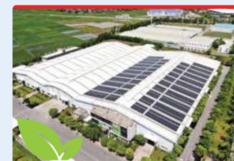
Tien Phong Plastic Factory project
